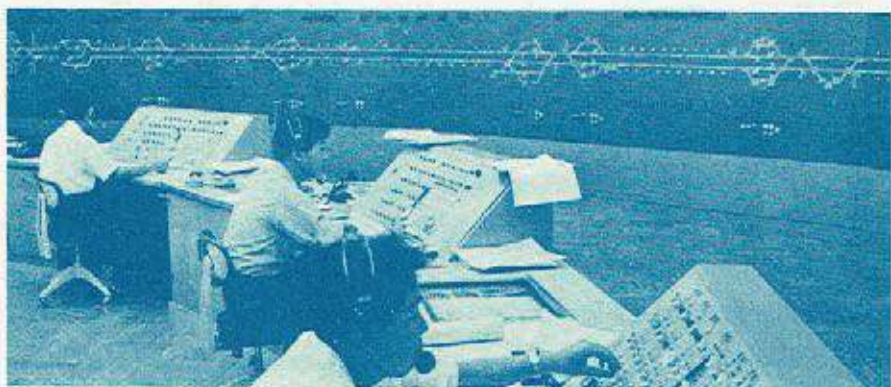
CENTRAL CONTROL CENTER. In the central dispatchers' room in Tokyo are control desks, equipped with signal levers for train control and with dispatching telephones. The panel on the wall shows the movements of all trains throughout the line.
