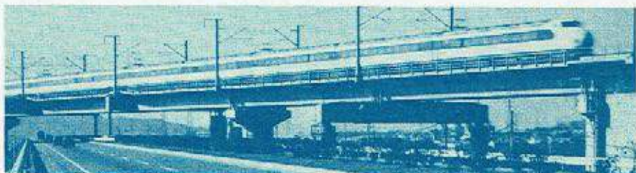
GRADE CROSSINGS. As a safety measure, there are no grade crossings on the New Tokaido Line. Much of the right-of-way is elevated above the surrounding terrain.
